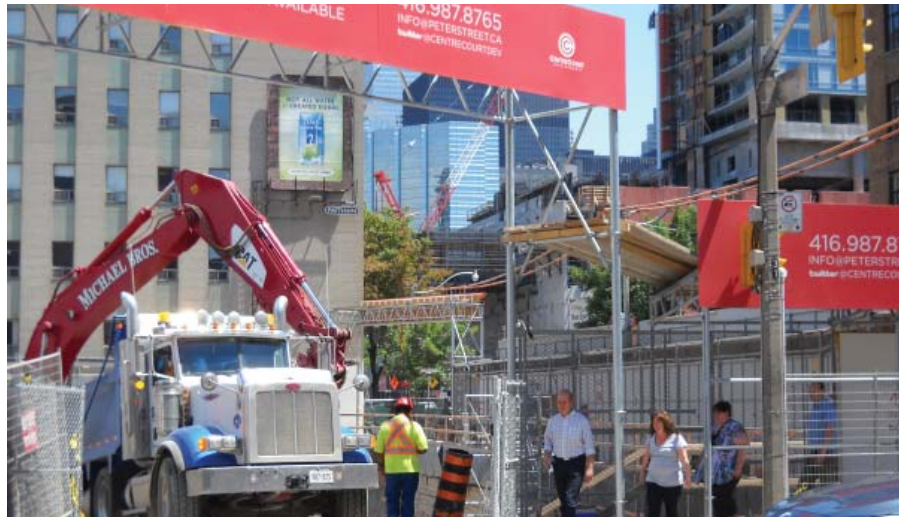
Construction begins at Peter Street Condos.
